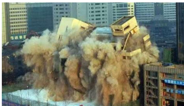
Figure 7. Demolition by blasting
